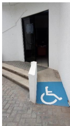
Rampa – D.I.F. Municipal
