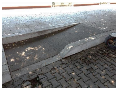
Rampa - Plaza Principal
